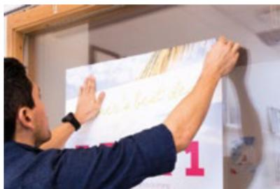
**3.** Use a soft sided "felt" squeegee to eliminate any air bubbles. Do not use of bubble popper tools or sharp objects to eliminate the bubbles.
